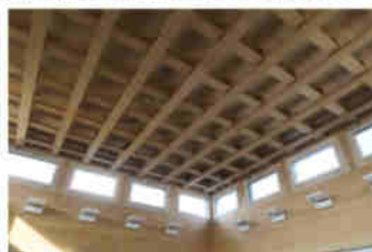
Deck des House of Natural Resources, THZ
