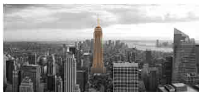
Metsä Wood and Michael Green have designed a wooden version of the Empire State Building
